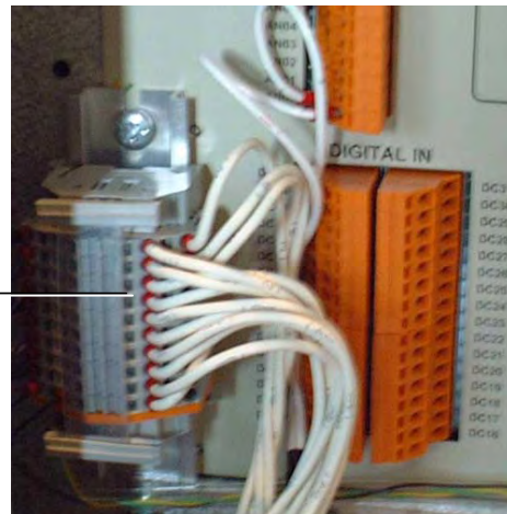
Dry contact connection to DC00 to DC51 (Using external power supply)
