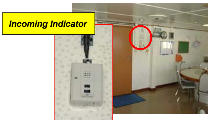
Fig. 5.4.5 Installation of BDE
