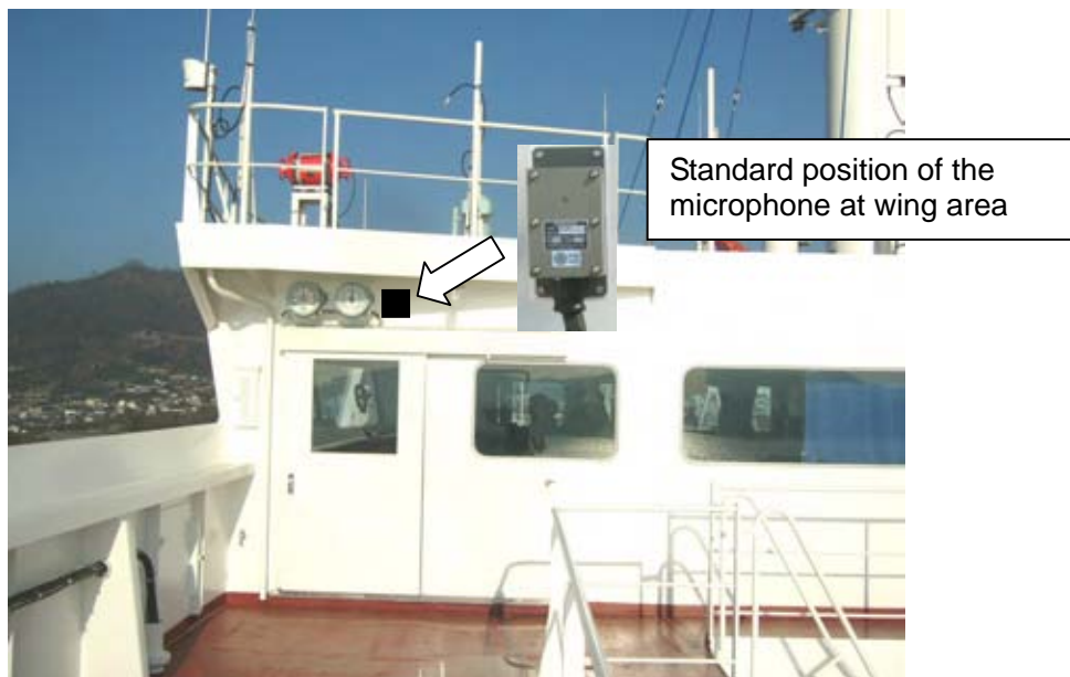
Fig. 9.2.6 Microphone installed in wing area-2
