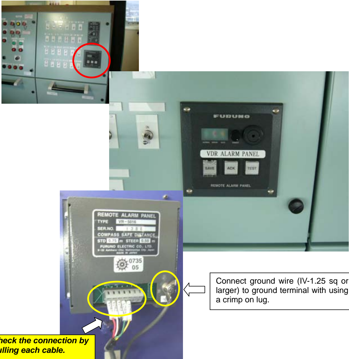
Fig. 9.2.1 Mounting of Remote Alarm Panel
