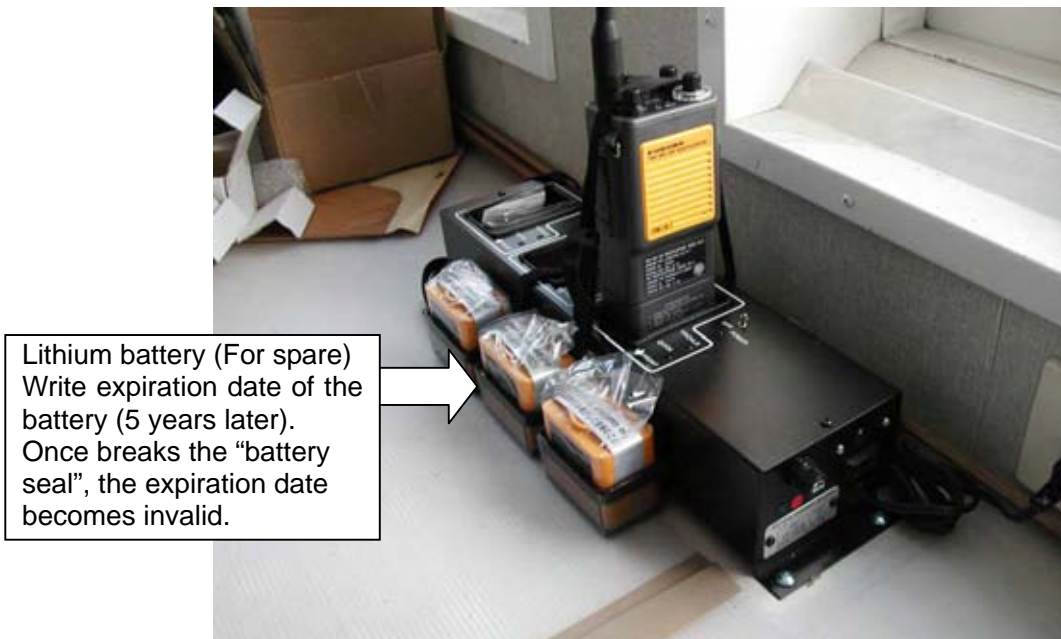
Fig. 10.2.2 Installation of Two-Way VHF Radio-2
