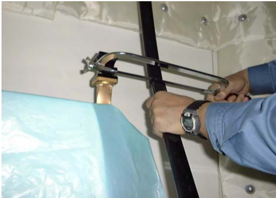
Fig. 1.2.21 Cutting wave-guide
