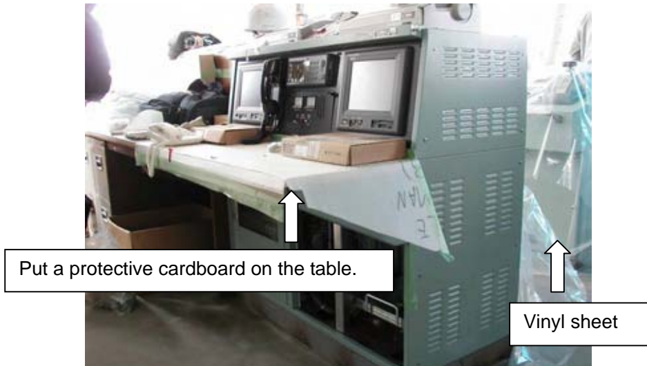
Fig. 3.3.1 Protect from damagingies
