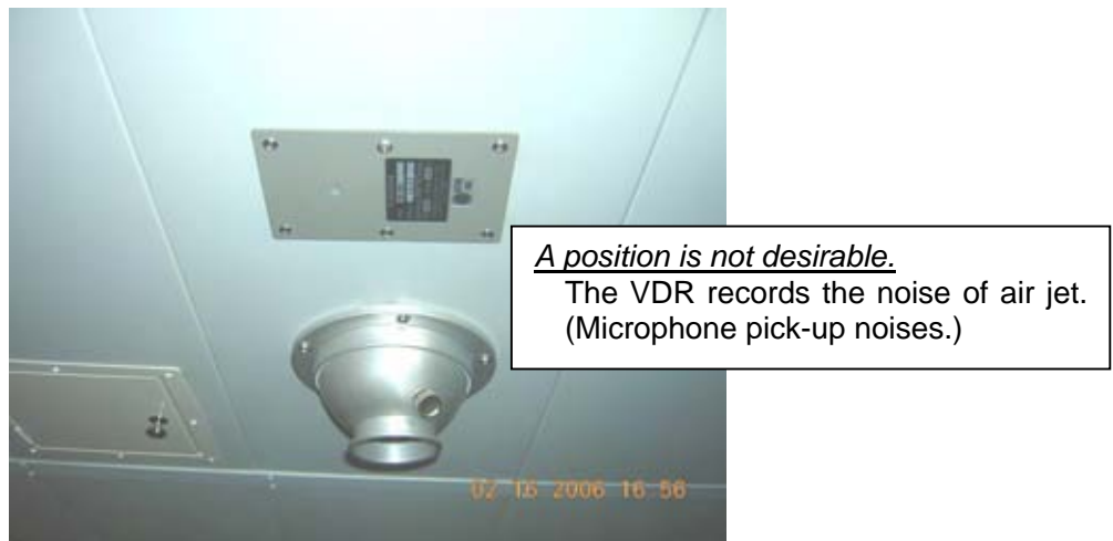
Fig. 9.2.4 Microphone installed in bridge-2
