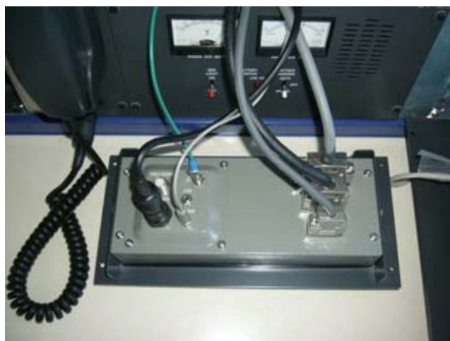
Fig. 3.3.13 Reassembling the terminal units
